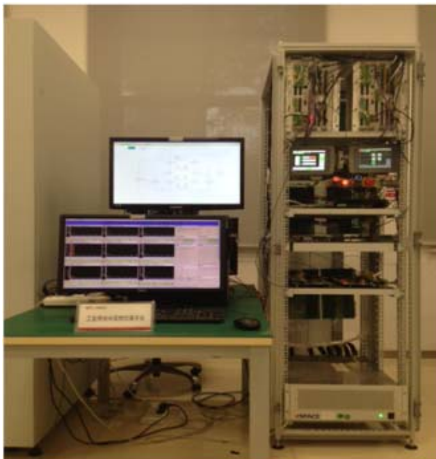
Fig. 9. Hardware-in-loop setup of the three-level medium-voltage transmission system.
