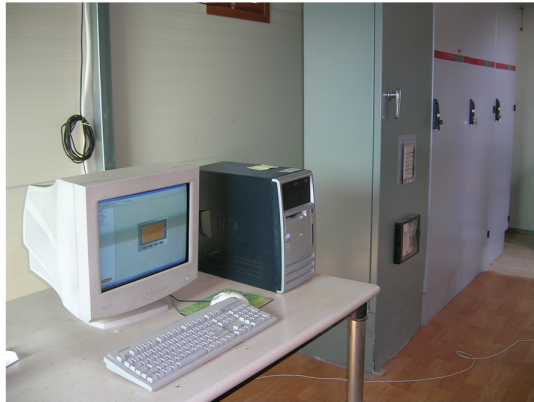
(b) Inverter groups of PV generation.
